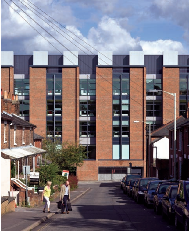
The old concrete facade (above) is broken up with external ducts clad in locally sourced brick (left).
